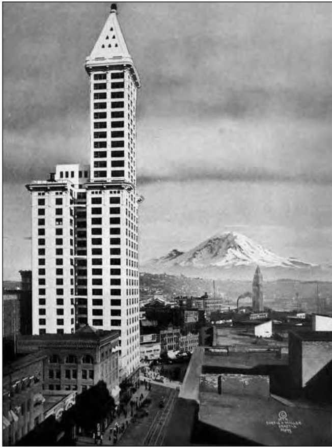
Smith Tower, Seattle, 1914. The King Street Station can be seen in the middle distance, and in the far distance, Mount Rainier.
